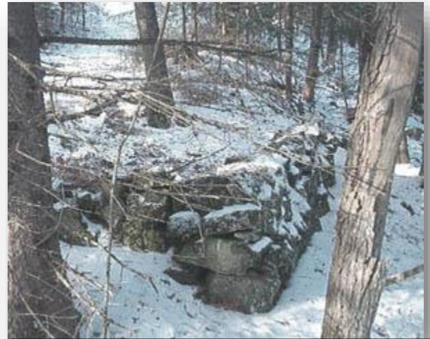
Small building foundation facing Ottawa River
